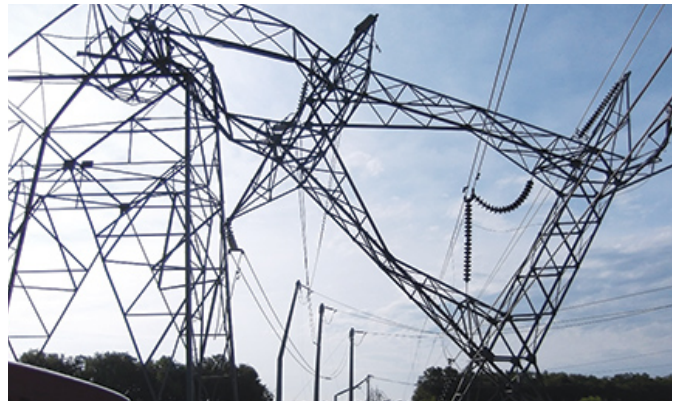
FIGURE 12: BENT LATTICE STRUCTURE SUPPORTED BY HPC
