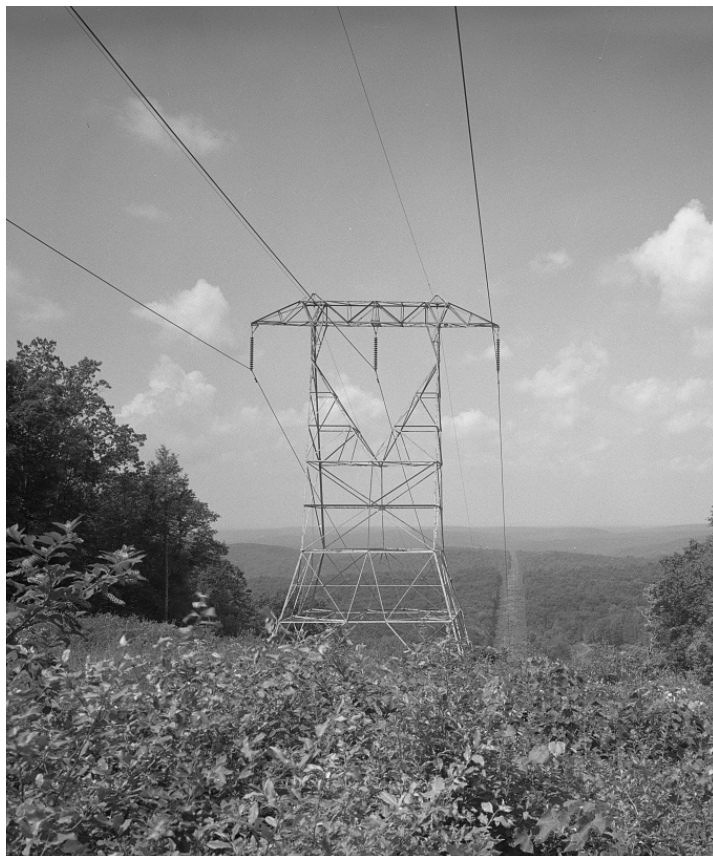
Figure 1 - A segment of the Roseland-Bushkill intertie in Stillwater. 45
