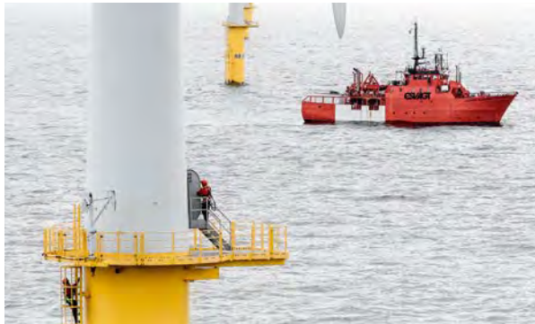
Credit: MHI Vestas Offshore Wind
